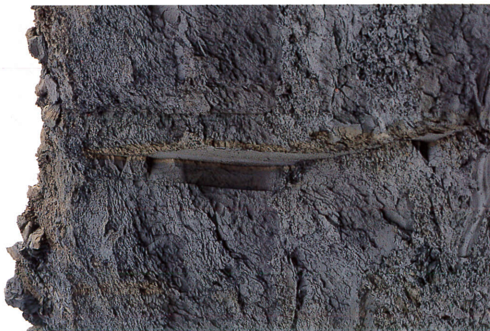
Photo 1 - Example of typical subvertical attitude of joints Castelnovo Berardenga quarry). In this case, as frequently happens, the fracture plane is grayish.
